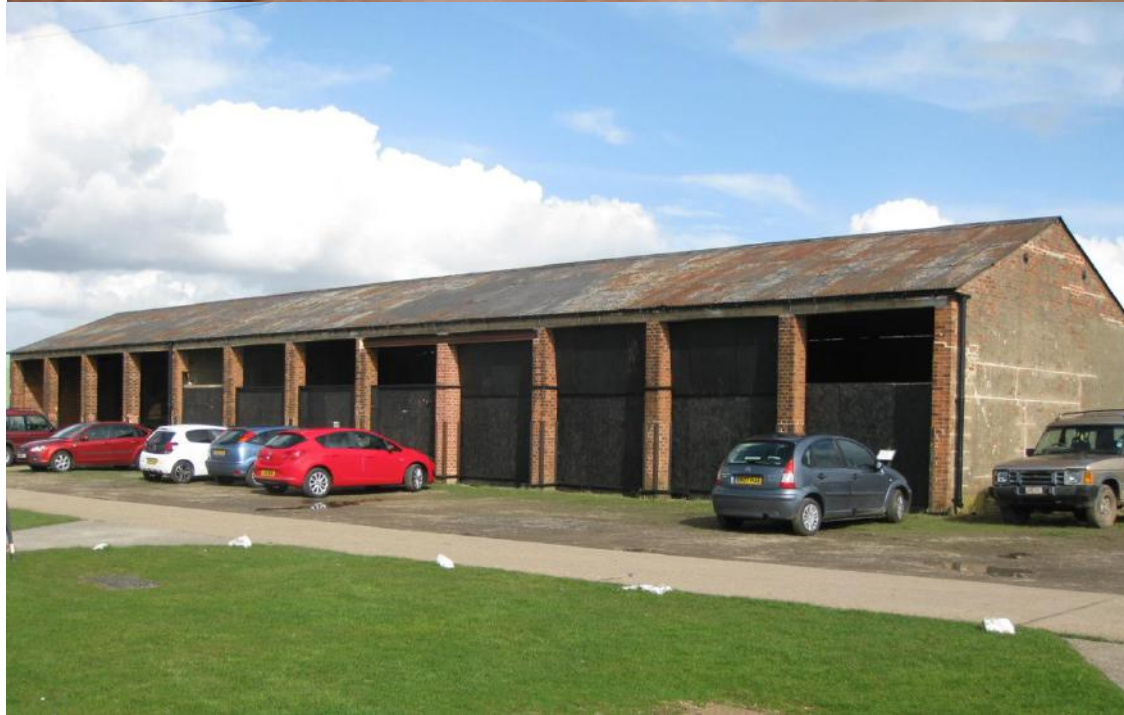
Stow Maries Aerodrome 'Tea at a Sports Day 1918' The building is the transport shed.
