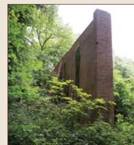
Back (west side) of the main brick wall.
