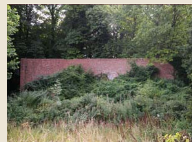
Front (east side) of the main brick wall.
